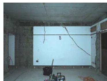
ひび割れ補修
